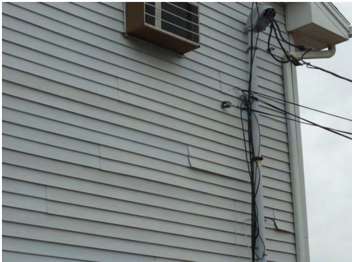
Typical vinyl siding repairs required.
