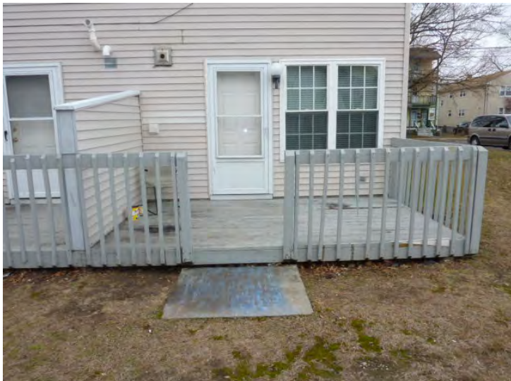
Typical rear wood porch in poor condition.
