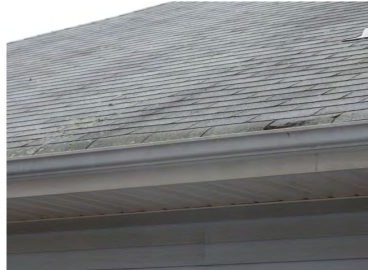
Typical worn and damaged roofing shingles.
