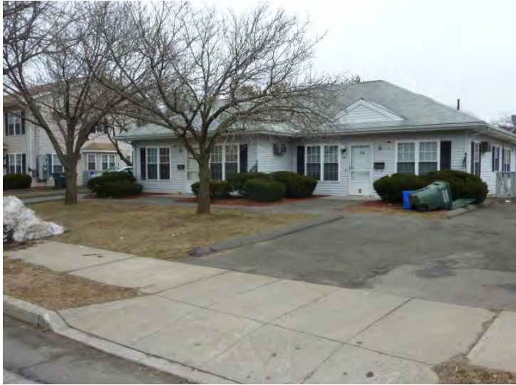
Asphalt driveways are in poor condition. Concrete walks are in generally good condition.
