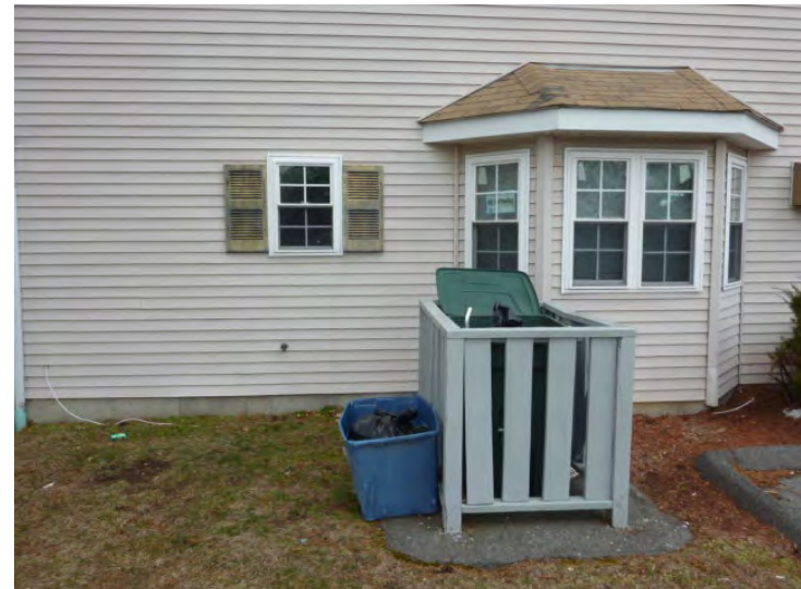
Typical side elevation with faded shutters, worn roofing shingles, and trash enclosure painted and in poor condition.
