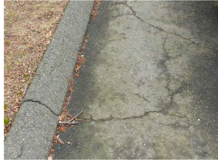
Typical cracking in asphalt paving site-wide.
